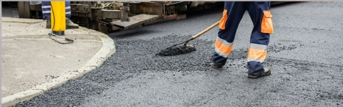
Construction and Maintenance of Streets and Infrastructure
