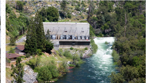
Kirkwood Powerhouse and Penstock
